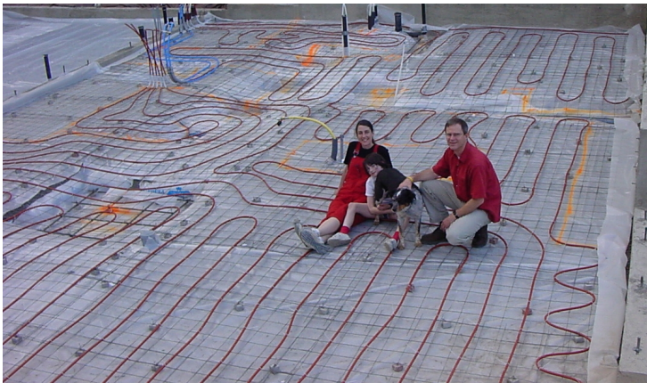
[Photo: Radiant floor PEX tubing installed before concrete was poured]
